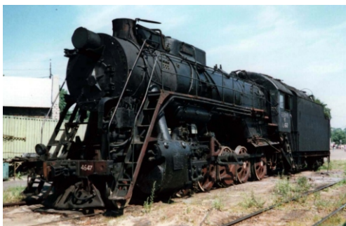
L Class decapod as a stationary boiler for laundry - Tallinn Steve Gould 1994
