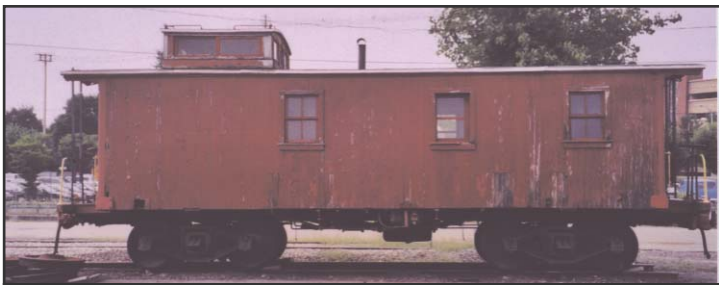
The north side of the caboose prior to removal of siding.
