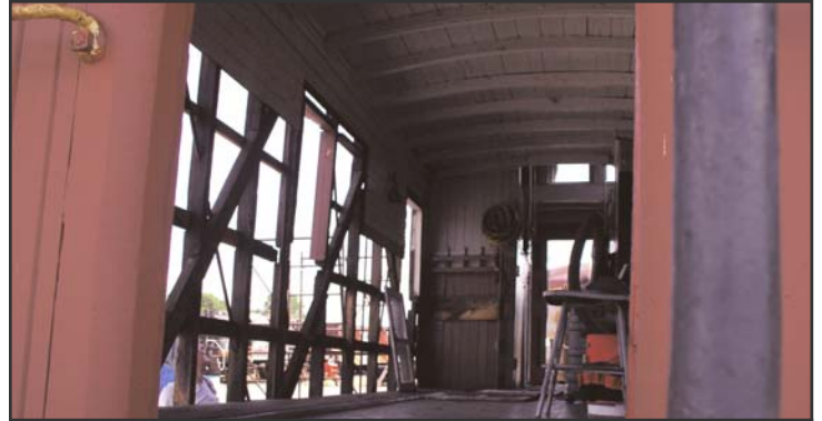
View of side from doorway prior to removal of framing.
